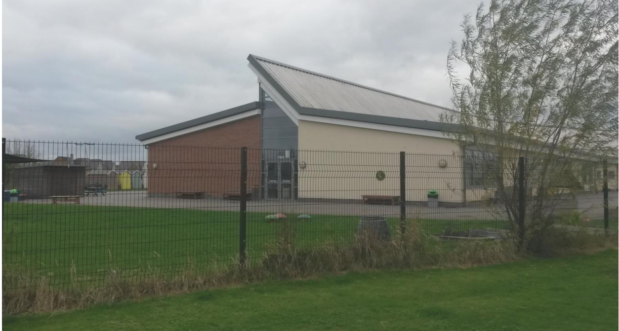
Existing eastern elevation of main building
