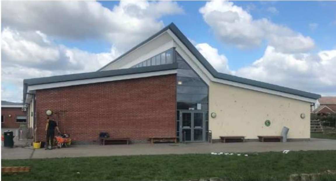
Existing building gable, location for new extension.
